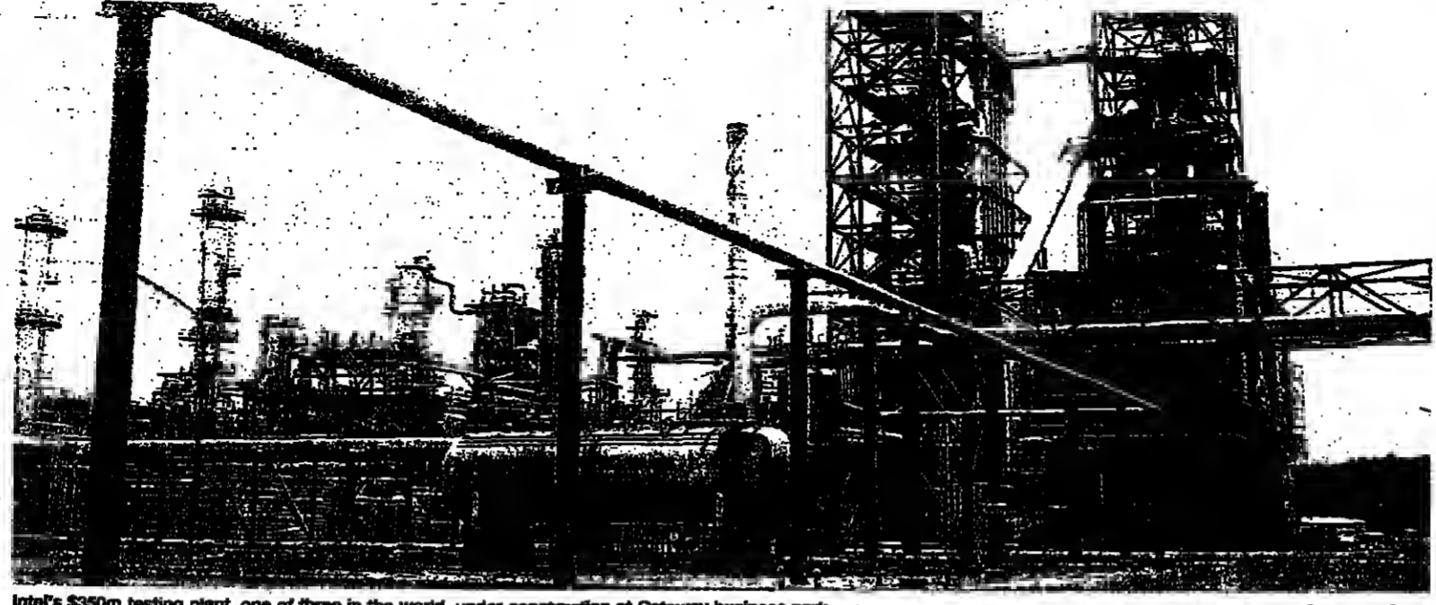
Intel's $350m testing plant, one of three in the world, under construction at Gateway business park.
